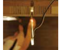
3/ Installation of the light appliance
