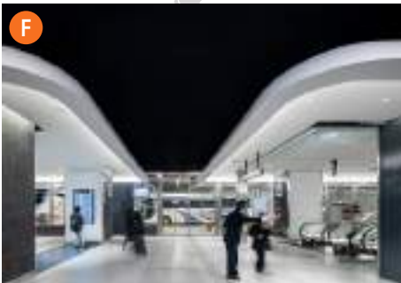
F Bus Terminal Tokyo Yaesu Location: Japan Creative Design Direction, Basic Design, Detailed Design: NIHON SEKKEI, INC. Detailed Design, Constructor: TAKENAKA CORPORATION Lighting design: NIHON SEKKEI, INC., LOOP LIGHTING, LLC Photo: ToLoLo studio
